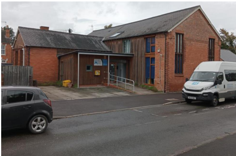
Existing building – principal (east) elevation to St Georges Walk
