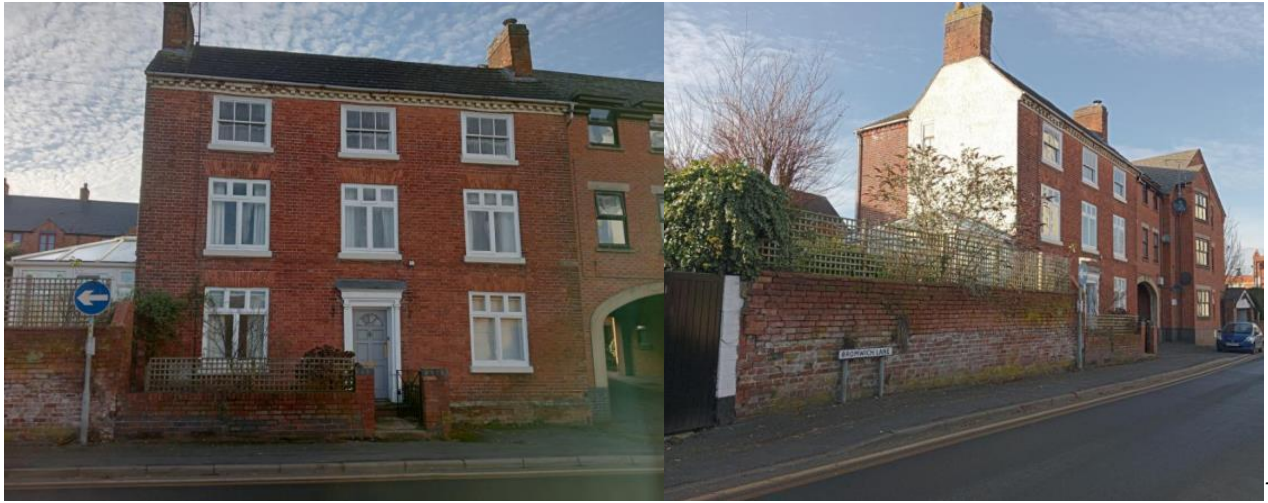
e application site, viewed from Bromwich Lane
