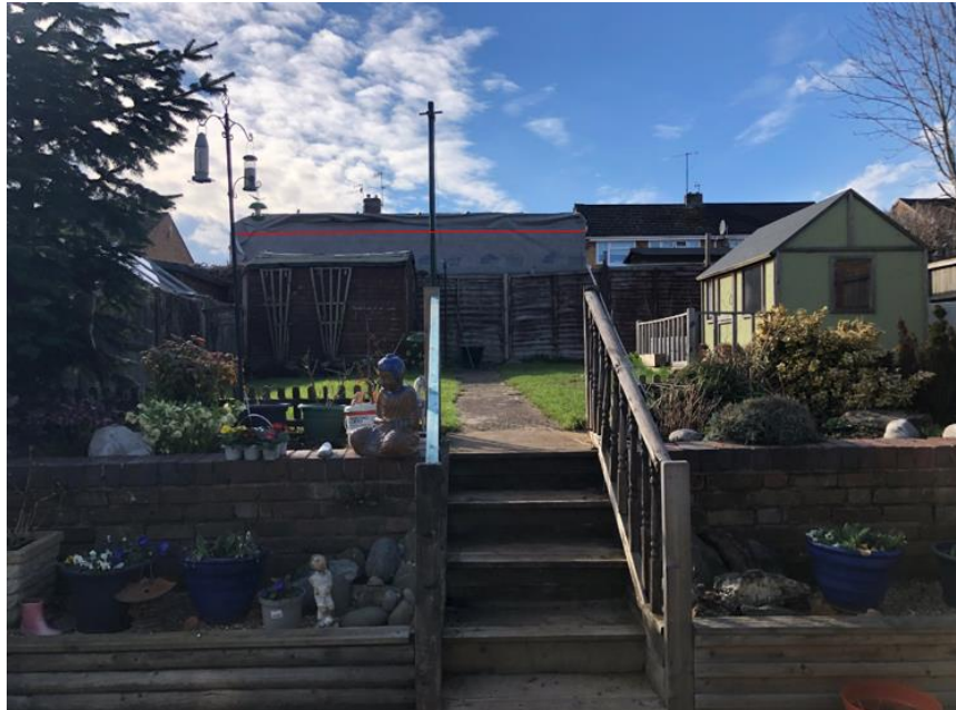
Figure 4 – Proposed building as erected (taken from the rear wall of the conservatory at 17 Sapphire Crescent)
