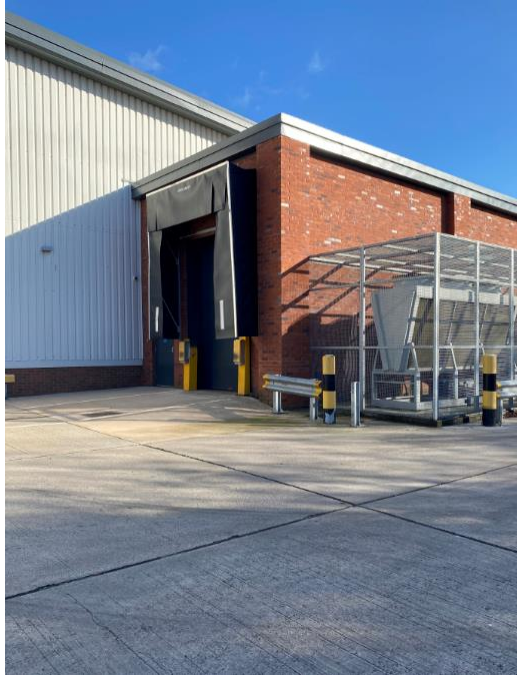
Figure 3 - Photograph showing the loading dock
